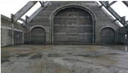
Ongoing Construction Project at St. Justin De Jacobis, St. Vincent De Paul Parish – Financed by Donholm Branch
